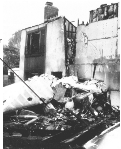
Figure 10 - The unbraced water heater in this home fell during an earthquake; the resulting fire destroyed the home.
