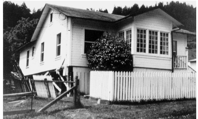
California Seismic Safety Commission
