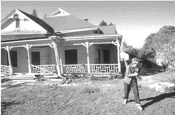
Figure 2 - Loma Prieta Earthquake, Oct. 17, 1989 Home moved off of its foundation and was considered a total loss.
