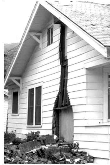
Figure 4 - Northridge Earthquake, Jan. 17, 1994 Chimney Collapse - common type of damage to unreinforced masonry.
